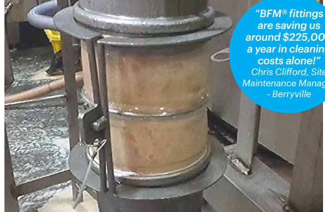
The snap-fit BFM® fitting system with the Tyson clamp
